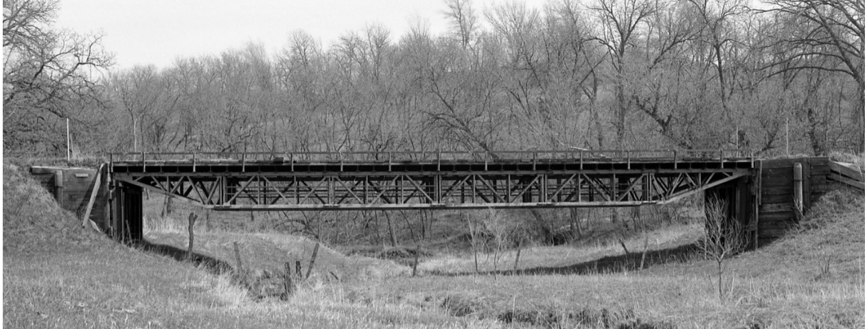
A photo taken in the 90s, looking west at structure.
