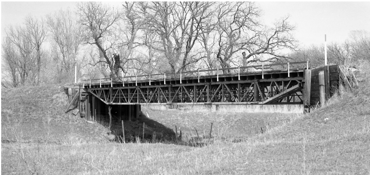
A photo taken in the 90s, looking northwest at structure.
