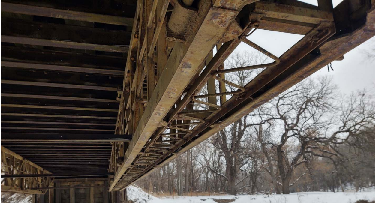
Present day photo, looking northeast at deck truss.
