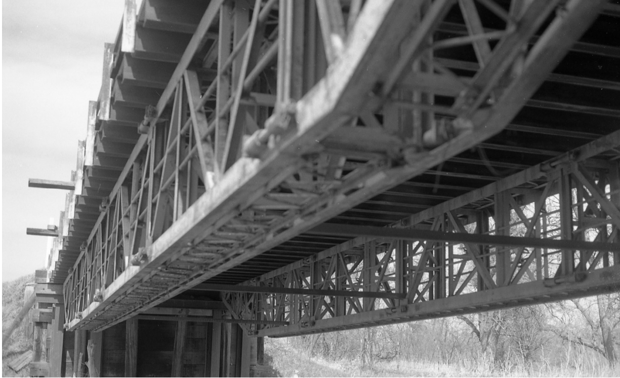
A photo taken in the 90s, looking northwest at deck truss.
