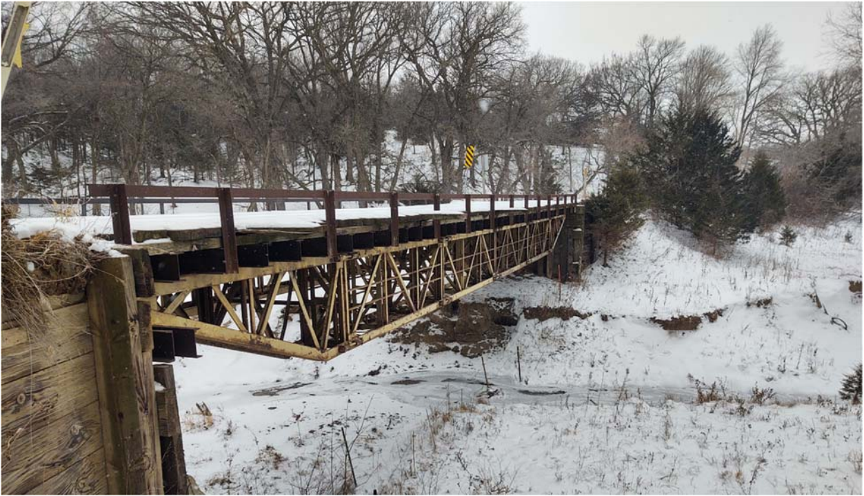
Present day photo, looking southeast at bridge.
