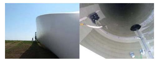
This blade is waiting to be attached. Note the curvature of the blade. The picture on the right is of the sensors inside the blade.
