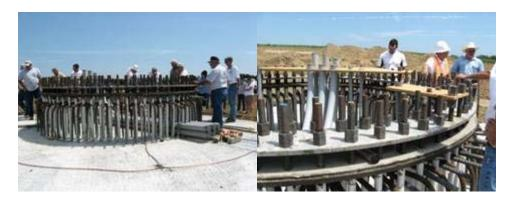
This shows the connections for the tower, conduit for the cabling, and the ground wire. The close up photo shows the bolts that will anchor the tower.
