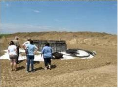
This is the base of a tower showing cement footings with the rebar. There are 48 tons of rebar and 495 cubic yards of cement per foundation.
