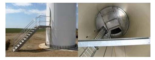
The base of the tower shows the large bolts anchoring it. Only a small portion of the cement is visible now.
