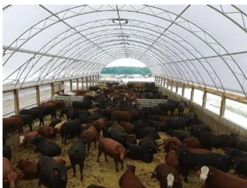
Example of a hoop building for livestock
