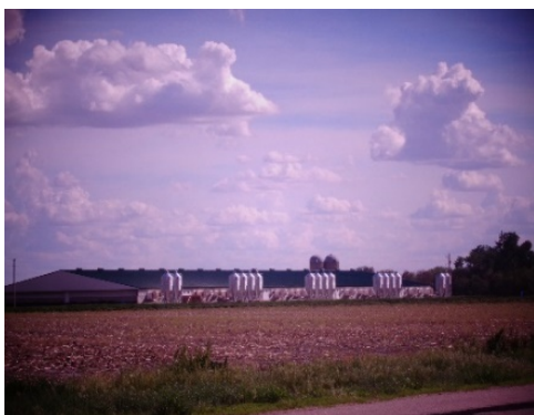
Example of an Animal Confinement Building
