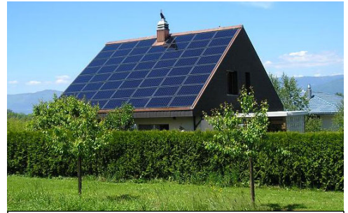
Example of a Solar Conversion System, Structure-mounted
