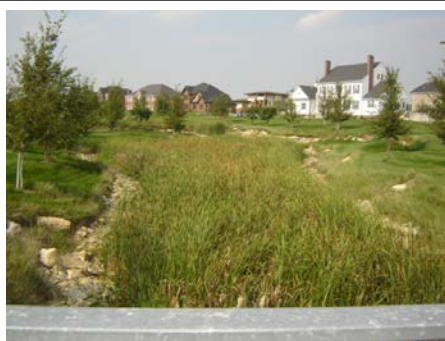
Example of a Drainageway or Surface Drain
